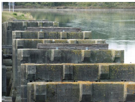
Fig. 3. Original concrete bridge supports on north side of bridge centre, re-surfaced with wooden sleepers taken from the old bridge trellis supports. Some concrete surface is still available on the resurfaced supports.
